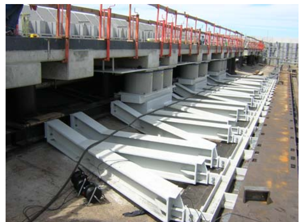
Figure 12: Framework after completion.
