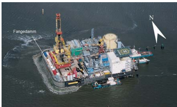
Figure 1: The drilling and mining platform „Mittelplate” in the state with the old drilling rig.
